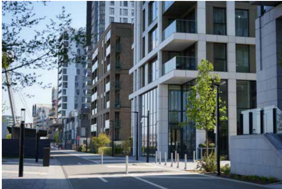
VIEW OF ADJACENT BUILDINGS
