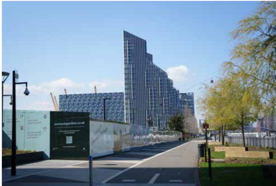
VIEW ALONG OLYMPIAN WAY
