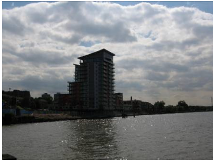
Photograph East of Phase 1 taken early evening
