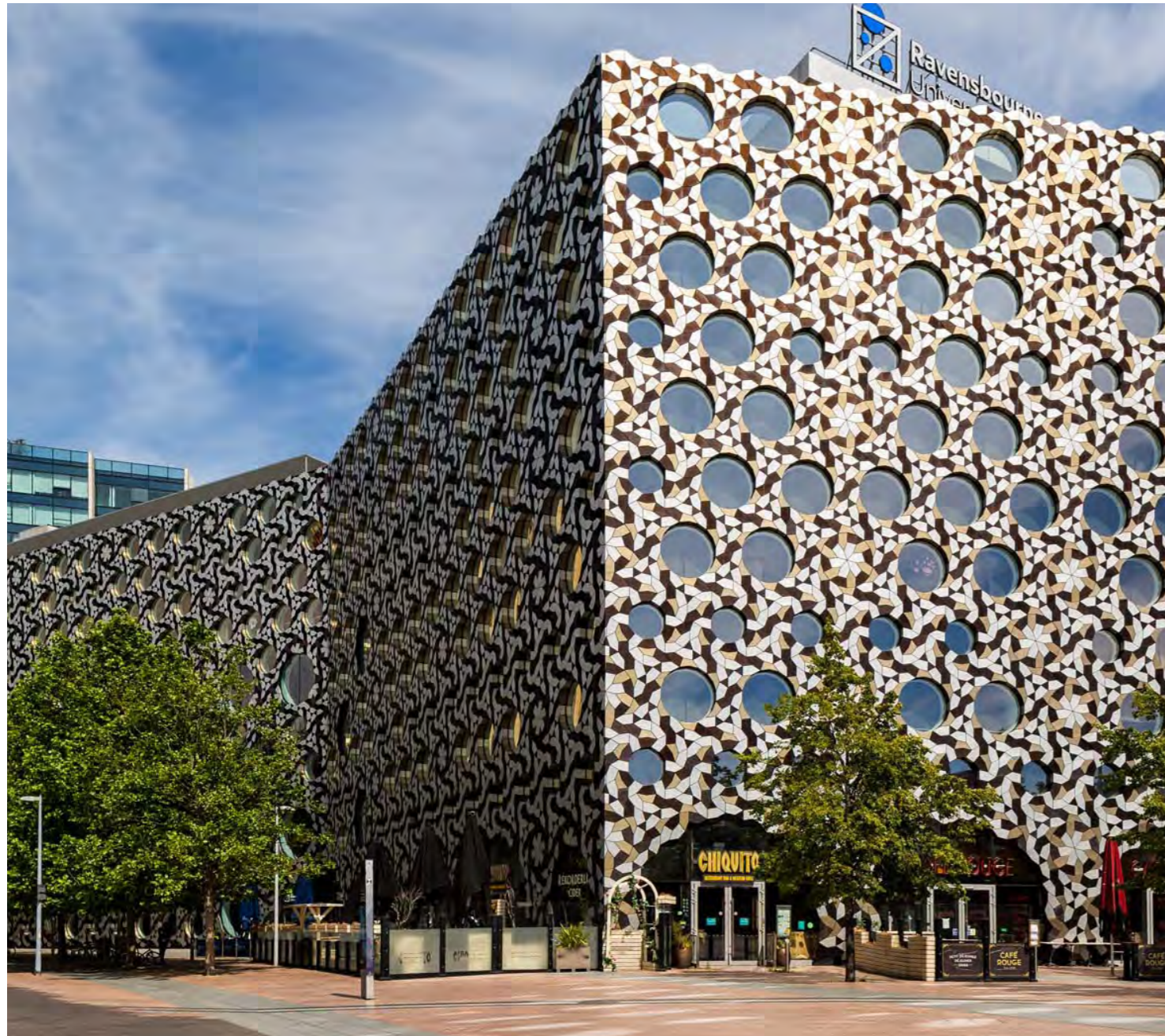
Ravensbourne College and offices
