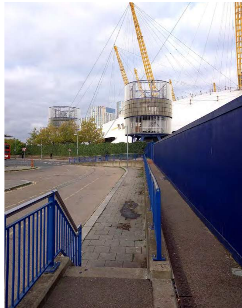
04 footpath to the west of the site
