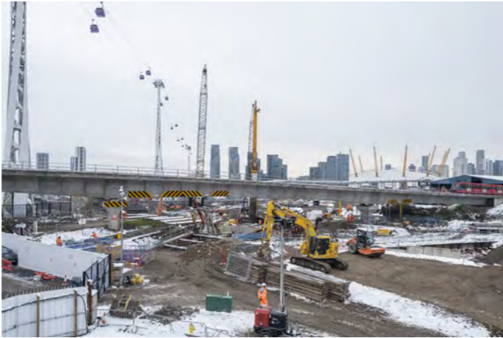
View 01 - Silvertown flyover
