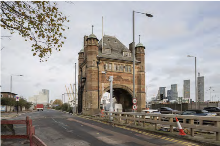
View 06 - Blackwall Tunnel Entrance Building
