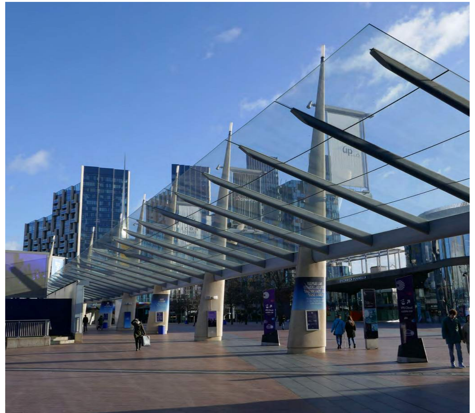
The O2 canopy + station entrance
