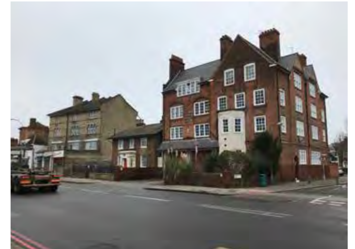
Figure 7.10 Lee Green Fire Station
