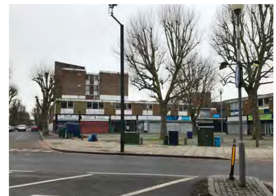
Figure 4.7 Looking south towards Leegate Centre from Eltham Road.
