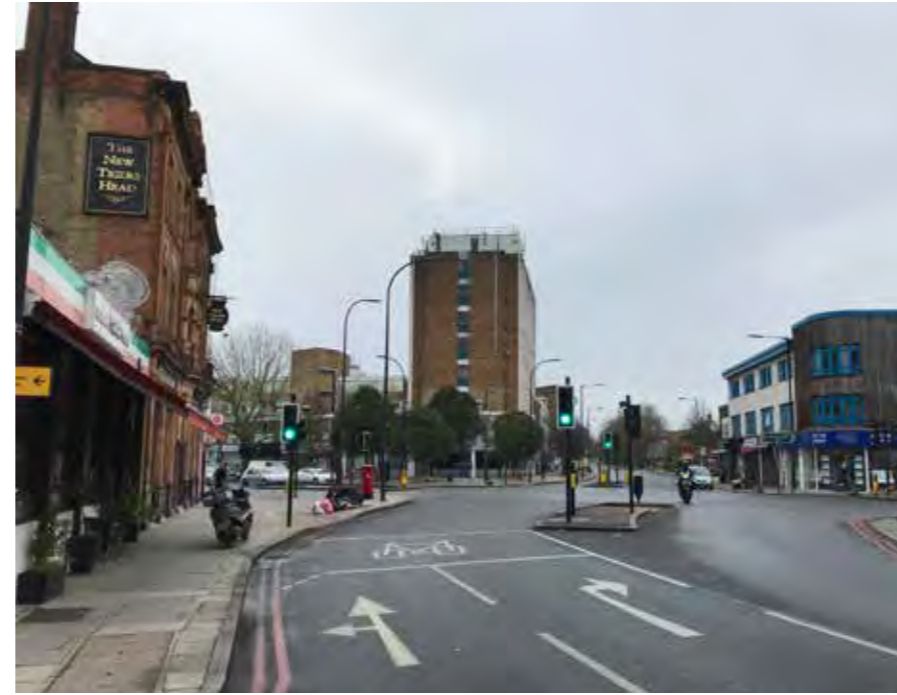
Figure 4.3 Looking south on Lee Road, towards Leegate House. The flank elevation of Leegate House faces the junction.
