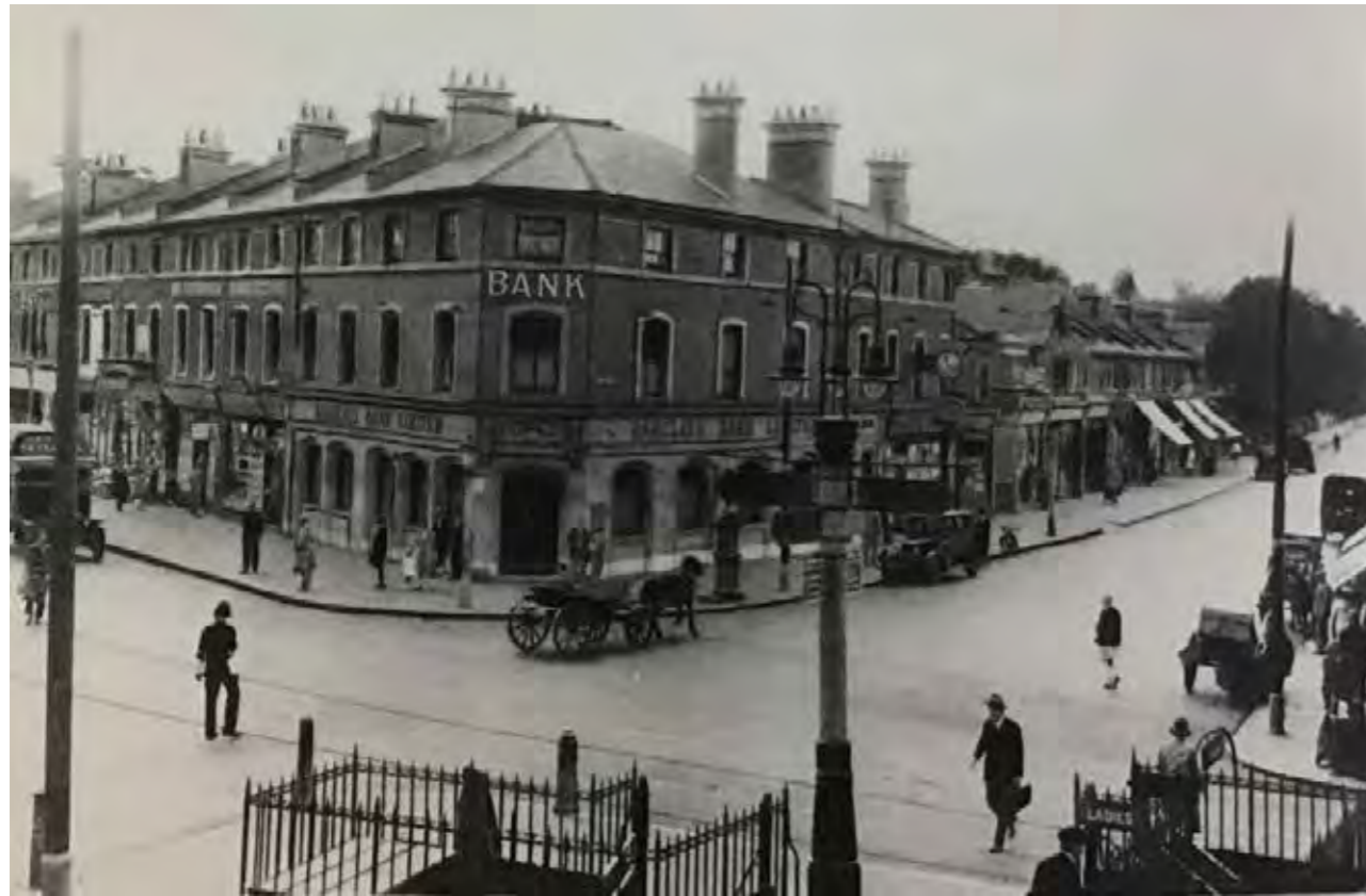
Figure 3.13 Looking from the Old Tiger's Head Pub south-east across the Lee Green junction towards Barclay's Bank. The bank and group of shops in this image are no longer occupied by the Leegate Centre.
