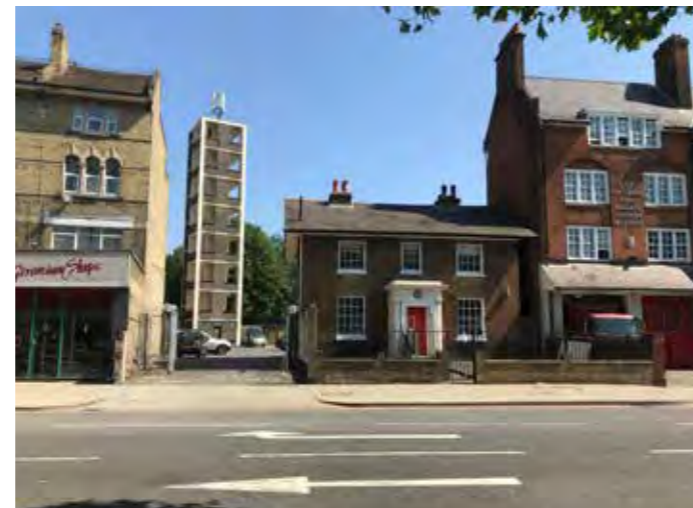
Figure 7.22 No. 7 Eltham Road (to the west - left - of the Fire Station)
