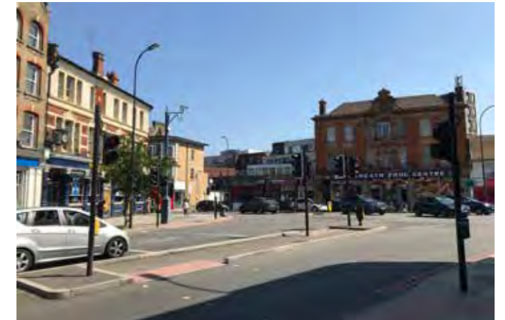
Figure 4.8 The Old and New Tiger's Heads Pubs (left and right) are the most prominent buildings on the north side of the Lee Green junction.
