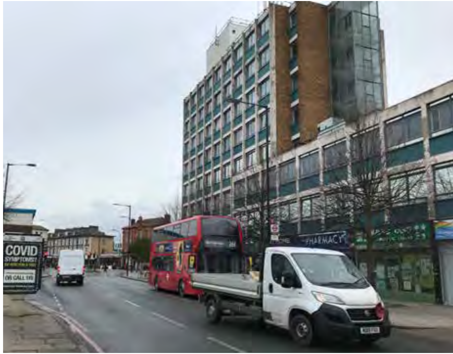
Figure 4.2 Leegate House, from Burnt Ash Road, looking south towards the junction.
