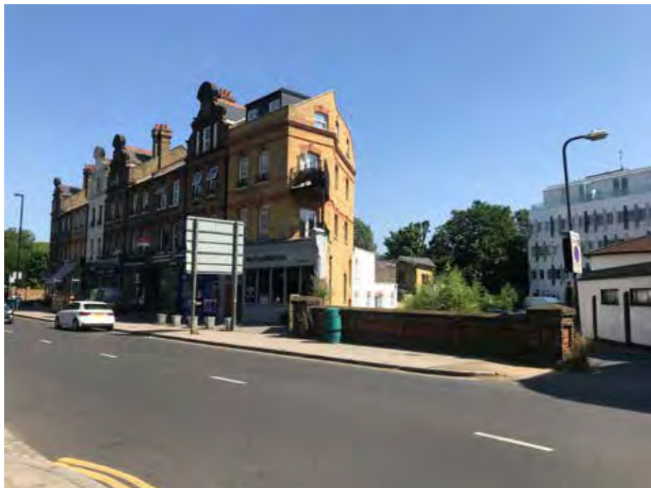
Figure 4.14 The River Quaggy cuts through under Lee Road, creating a break in the street-scape.
